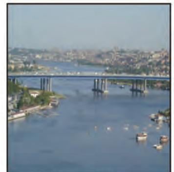
Haliç Bridge - (IHI Co-operation) Blasting & painting works
