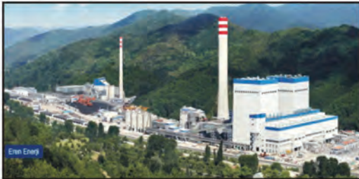
Eren Energy Thermoelectric Power plant - Blasting & coating - painting works
