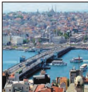
STFA - Galata Bridge Blasting & painting works
