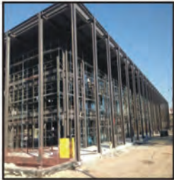
Abdullah Gül University Project 3000 tonnes of steel work and 40.000 m 3 blasting & painting works
