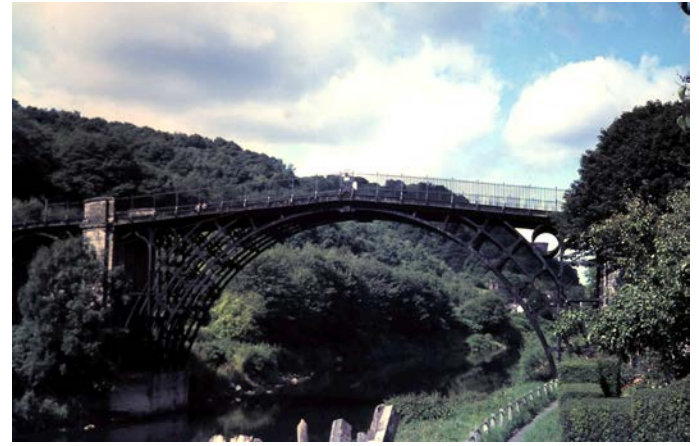
Iron Bridge Telford 1970 @ Gordon Spicer
